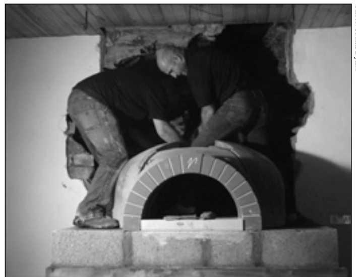
Installing the wood fired oven.
